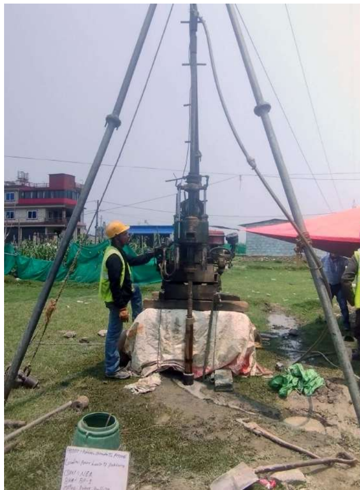
Drilling a Hole by Rotary Drilling Method (BH - 1 & AP - 1)
