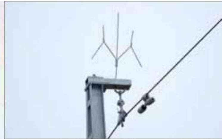
Wishbone Prevents Bird Landing on Wire
