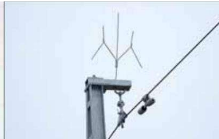
Wishbone Prevents Bird Landing on Wire
