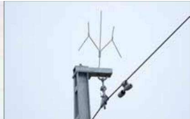
Wishbone Prevents Bird Landing on Wire
