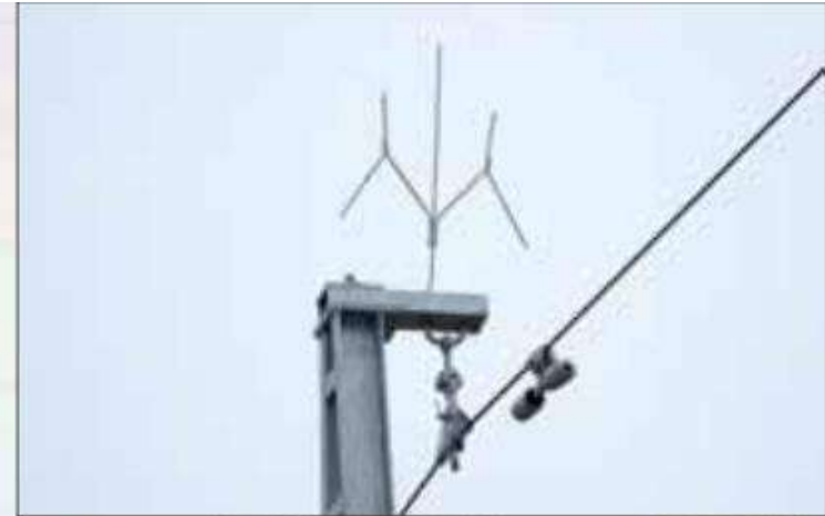
Wishbone Prevents Bird Landing on Wire
