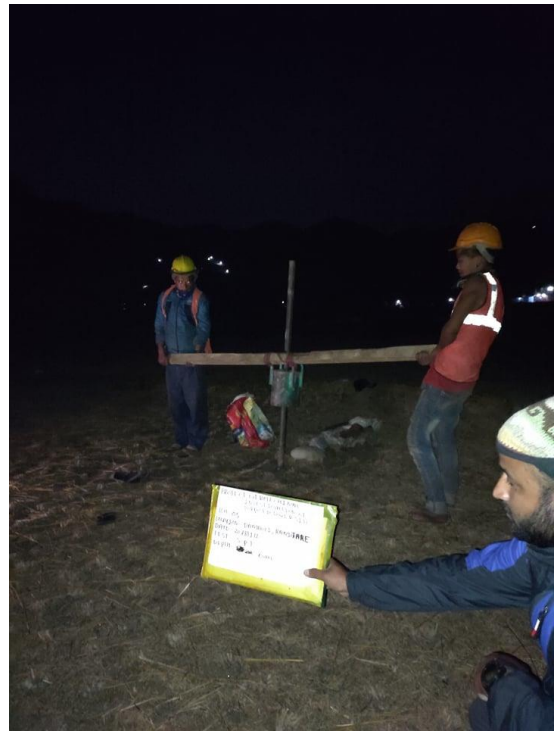
Conduction of Standard Penetration Test at Depth 4.5 m
