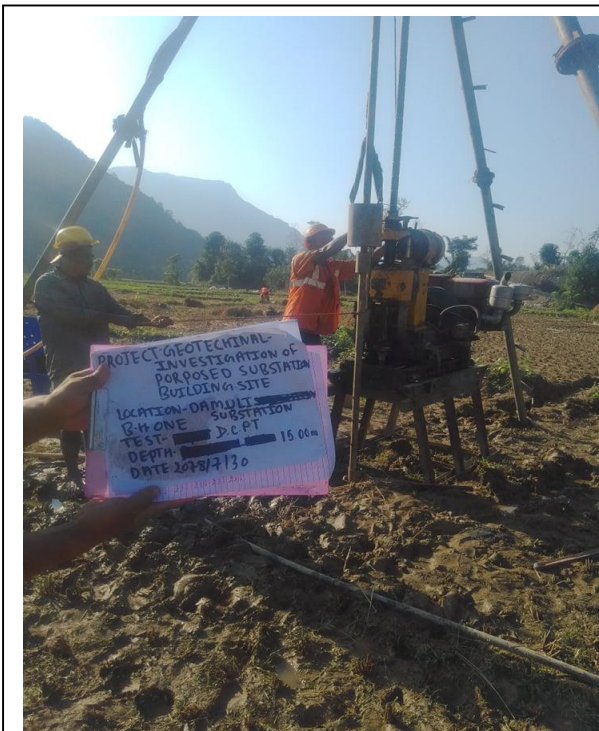
Conduction of Dynamic Cone Penetration Test at Depth 15.0 m
