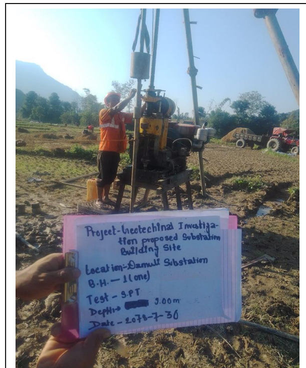
Conduction of Standard Penetration Test at Depth 9.0 m
