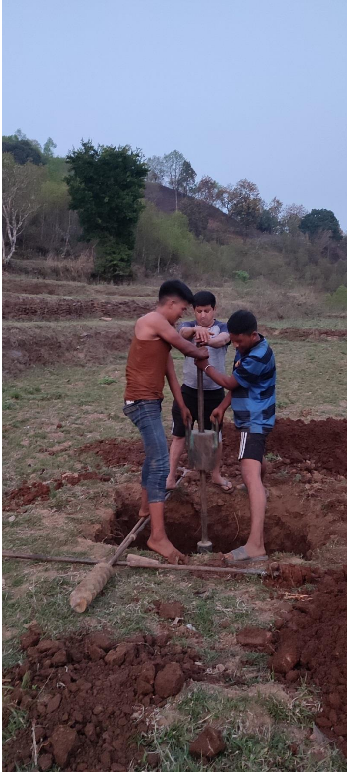
Conduction of Standard Penetration Test in Transmission Tower BH 3
