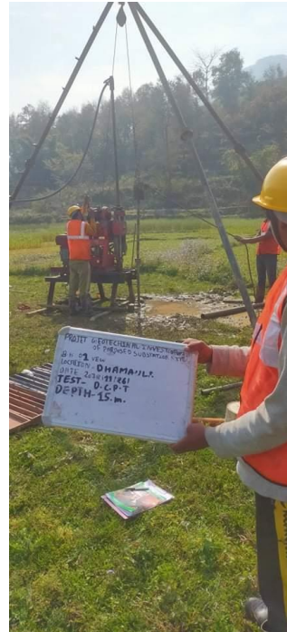
Conduction of Dynamic Cone Penetration Test at New Borehole 1 of Damauli SS; Depth 15 m
