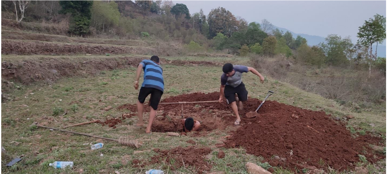
Augering in Process in Transmission Tower BH 3
