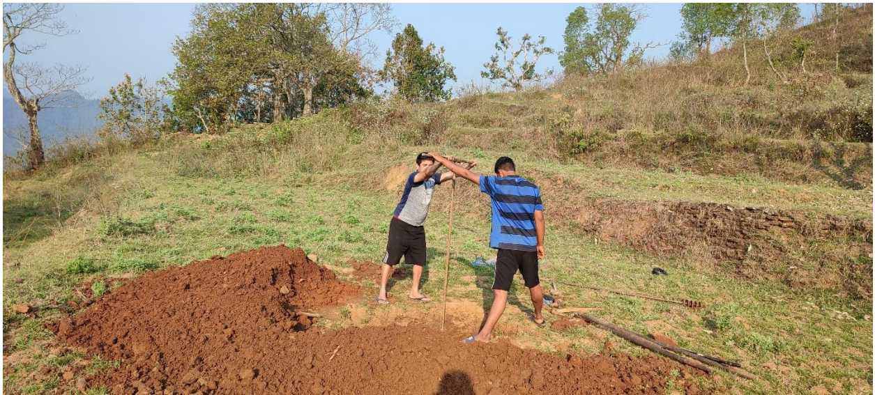
Augering in Process in Transmission Tower BH 3
