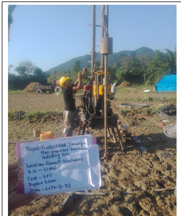
Conduction of Dynamic Cone Penetration Test at Depth 6.0 m
