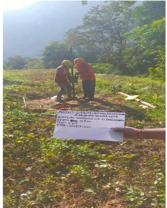
Conduction of Standard Penetration Test at Depth 4.5 m
