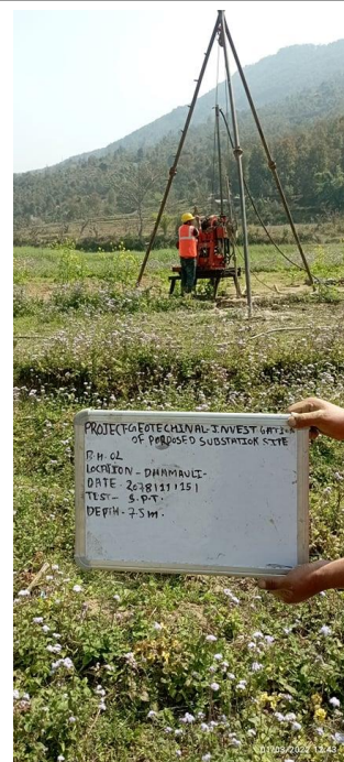
Conduction of Standard Penetration Test at New Borehole 2 of Damauli SS; Depth 7.5 m
