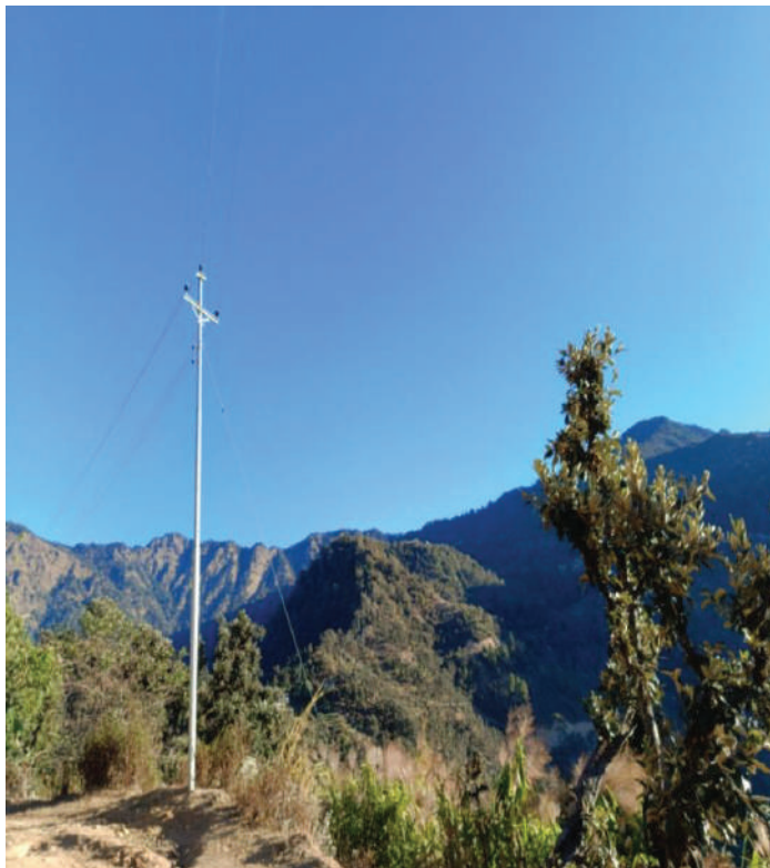
HT Line Extension work at Dailekh
