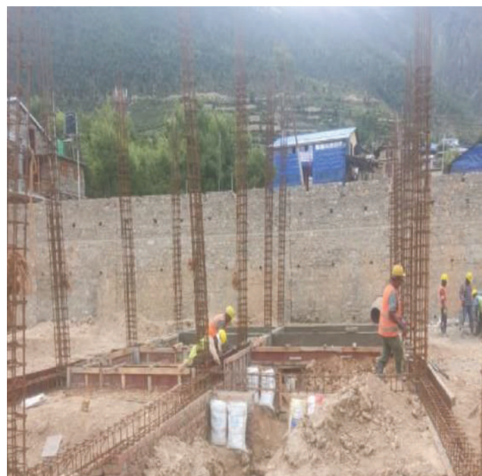
Ongoing Construction work at Simikot (Humla) S/S
