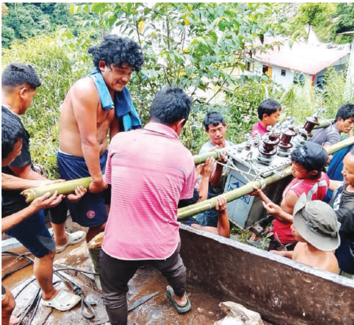
Transportation of distribution transformer by locals in Sankhuwasabha District
