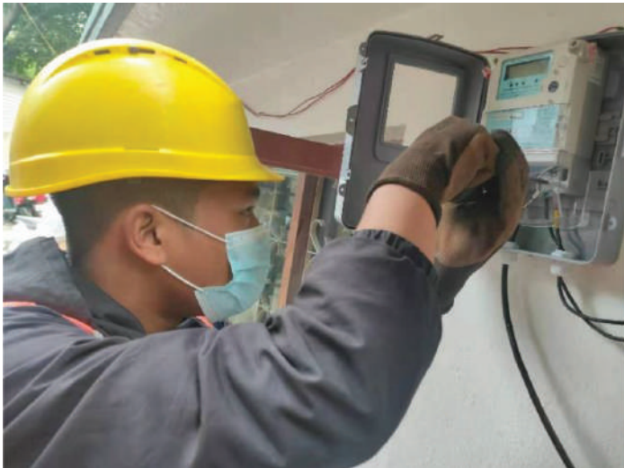
Installation of Smart Meter at Residential Consumer
