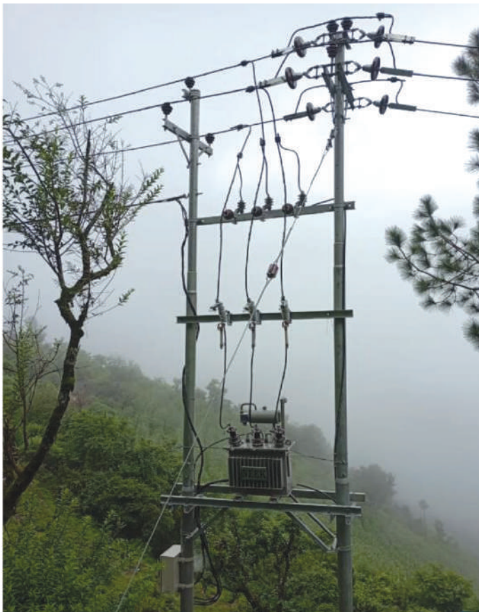
Line Erection works at Darchula District
