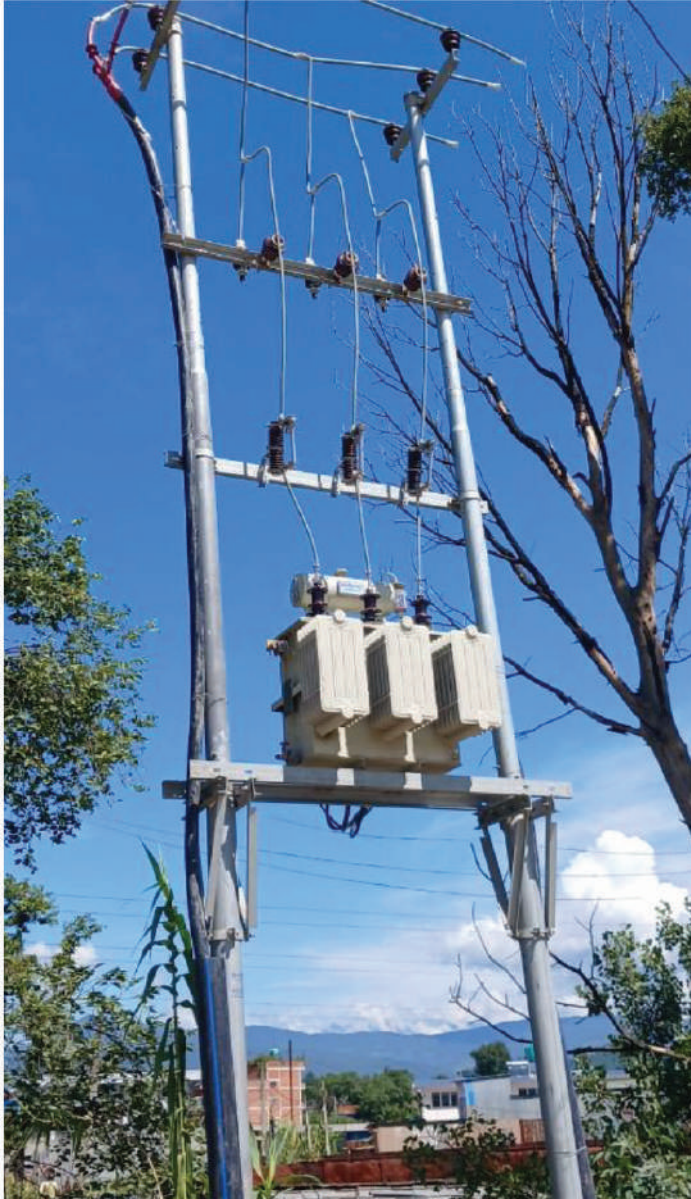
Installation of New DTR
