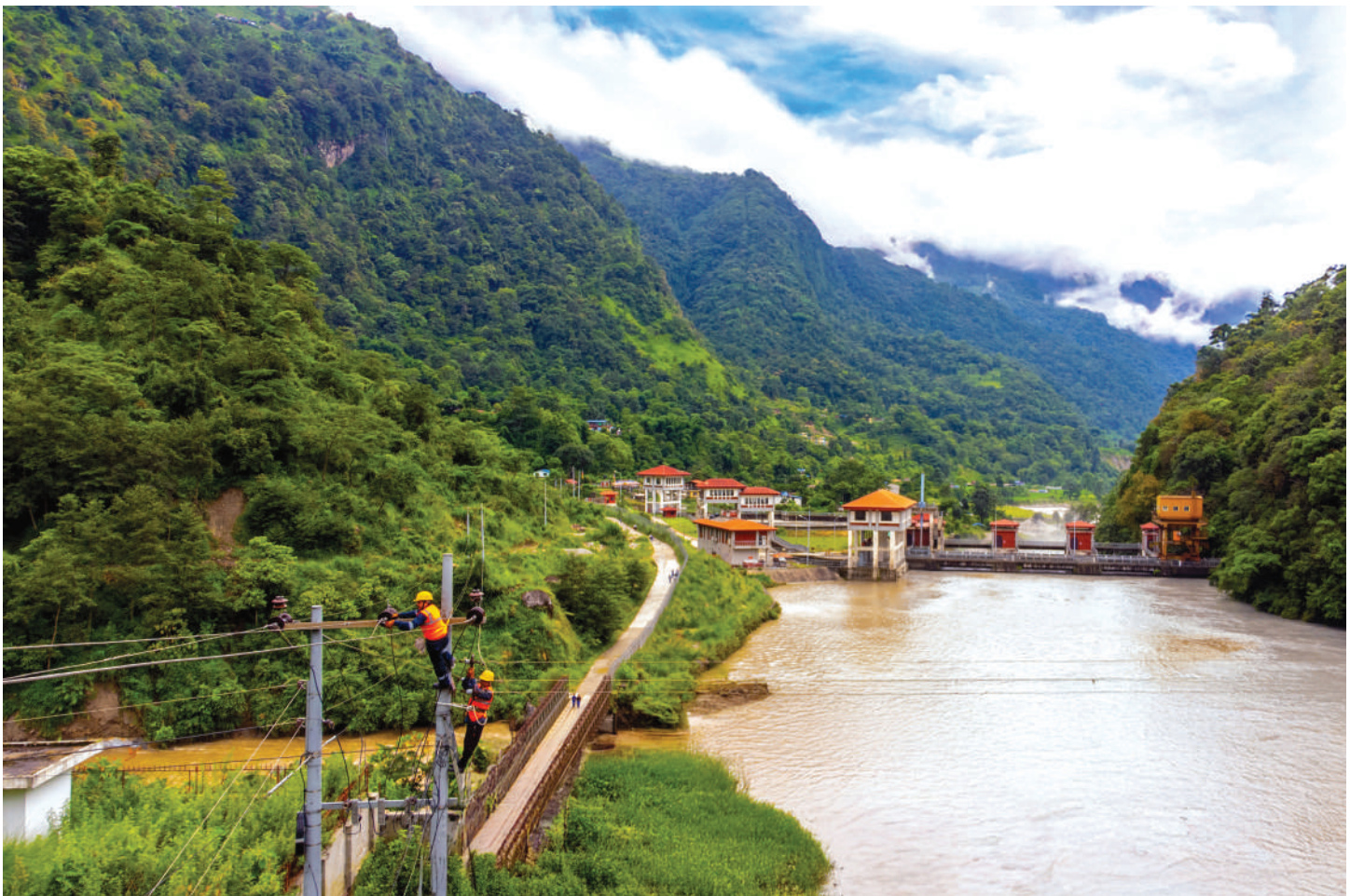
Line maintenance works at Lamjung DC
