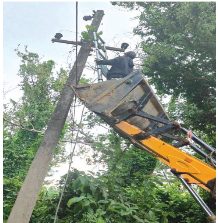
Repair and Maintenance works, Lumbini Province Division Office
