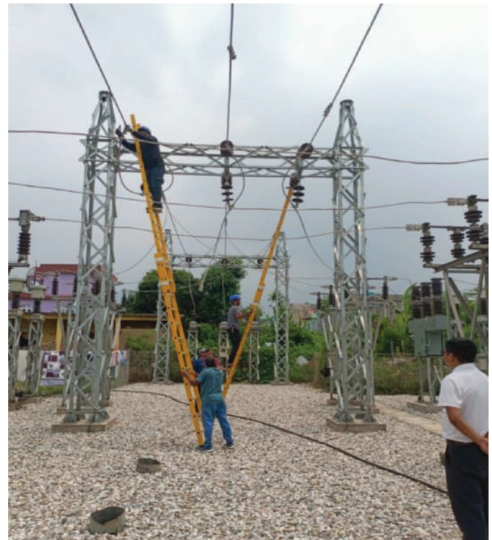
Maintenance work on 33/11kV Budbude Substation, Surkhet
