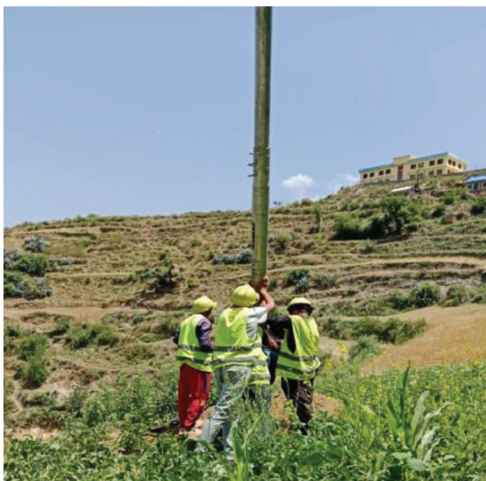
Erection of Pole at Mugu District
