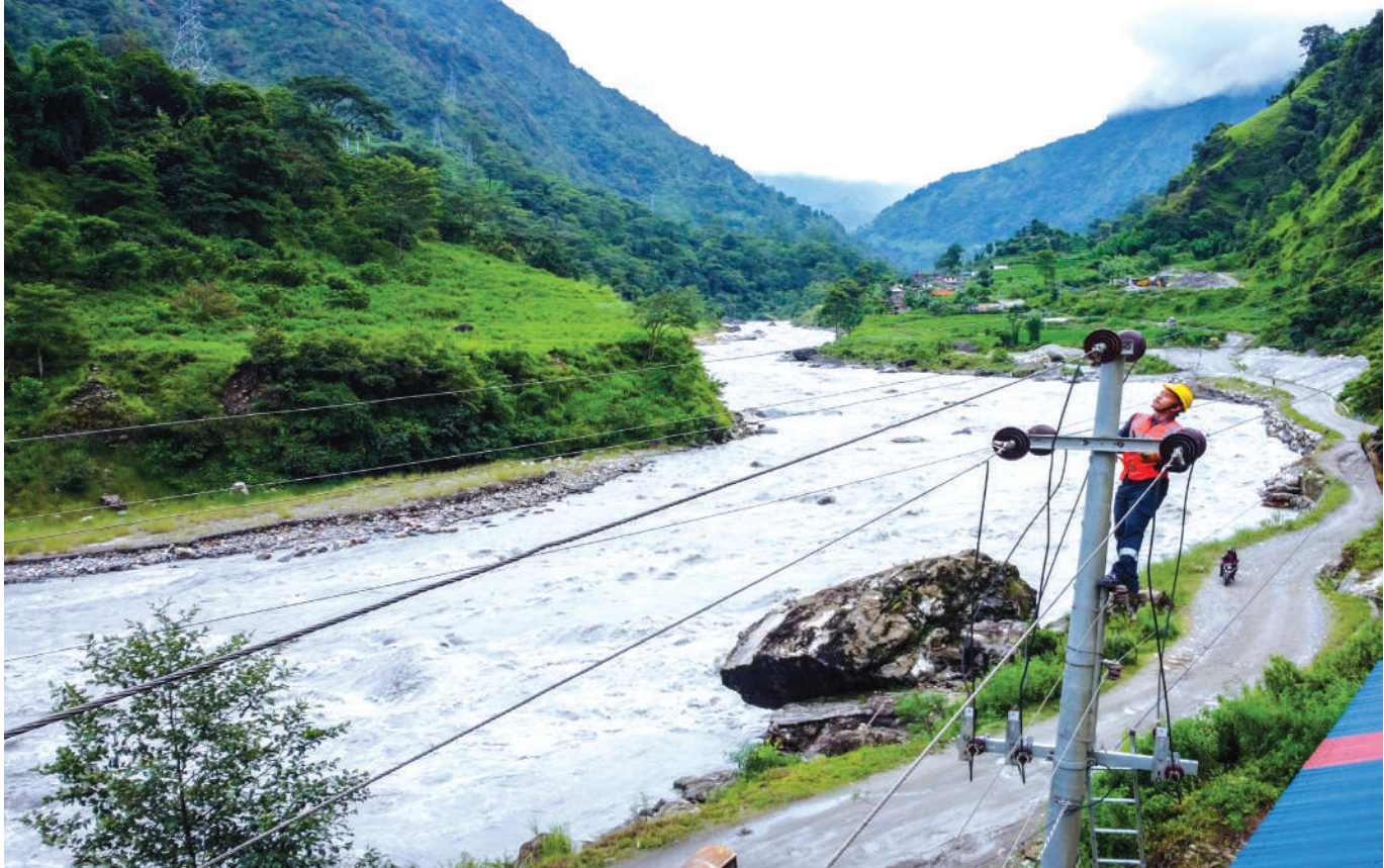
11 kV line maintenance works in Bhulbhule, Lamjung District
