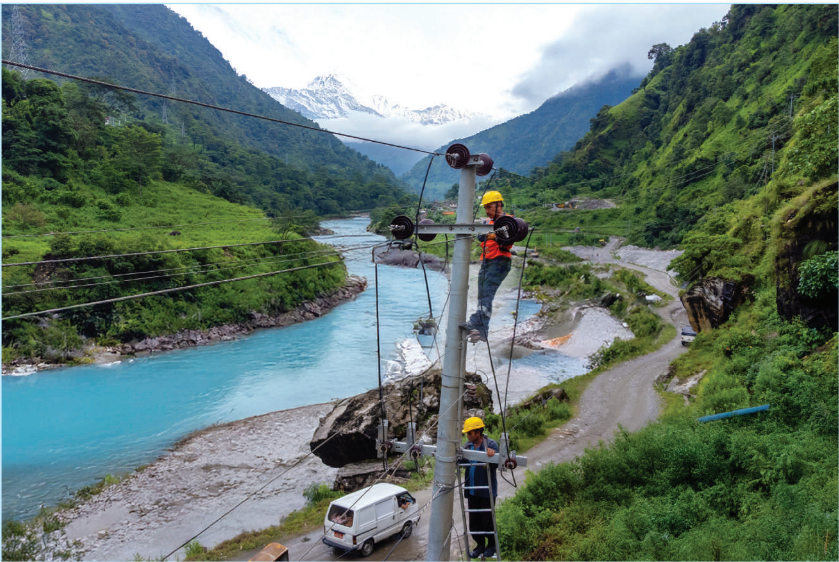
11 kV line maintenance works in Bhulbhule, Lamjung District
