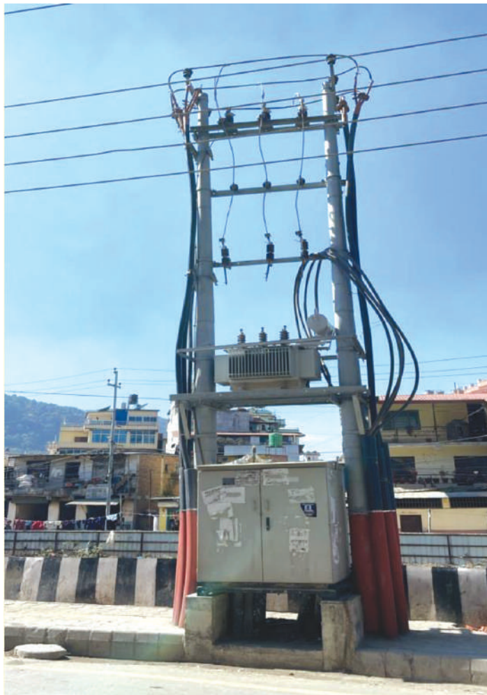
Installation of Distribution Transformer for commissioning of Underground Network.
