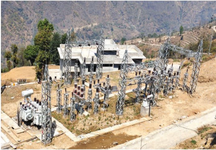
Underconstruction 33/11 kV, 8 MVA Jharlang substation, Dhading
