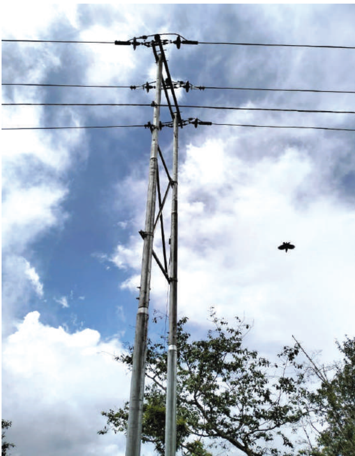
11 kV line extension works in Bhojpur District
