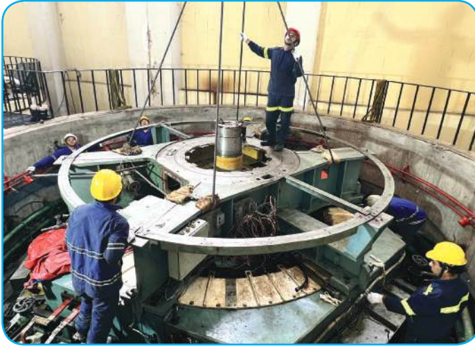
Dismantling of Generator bracket
