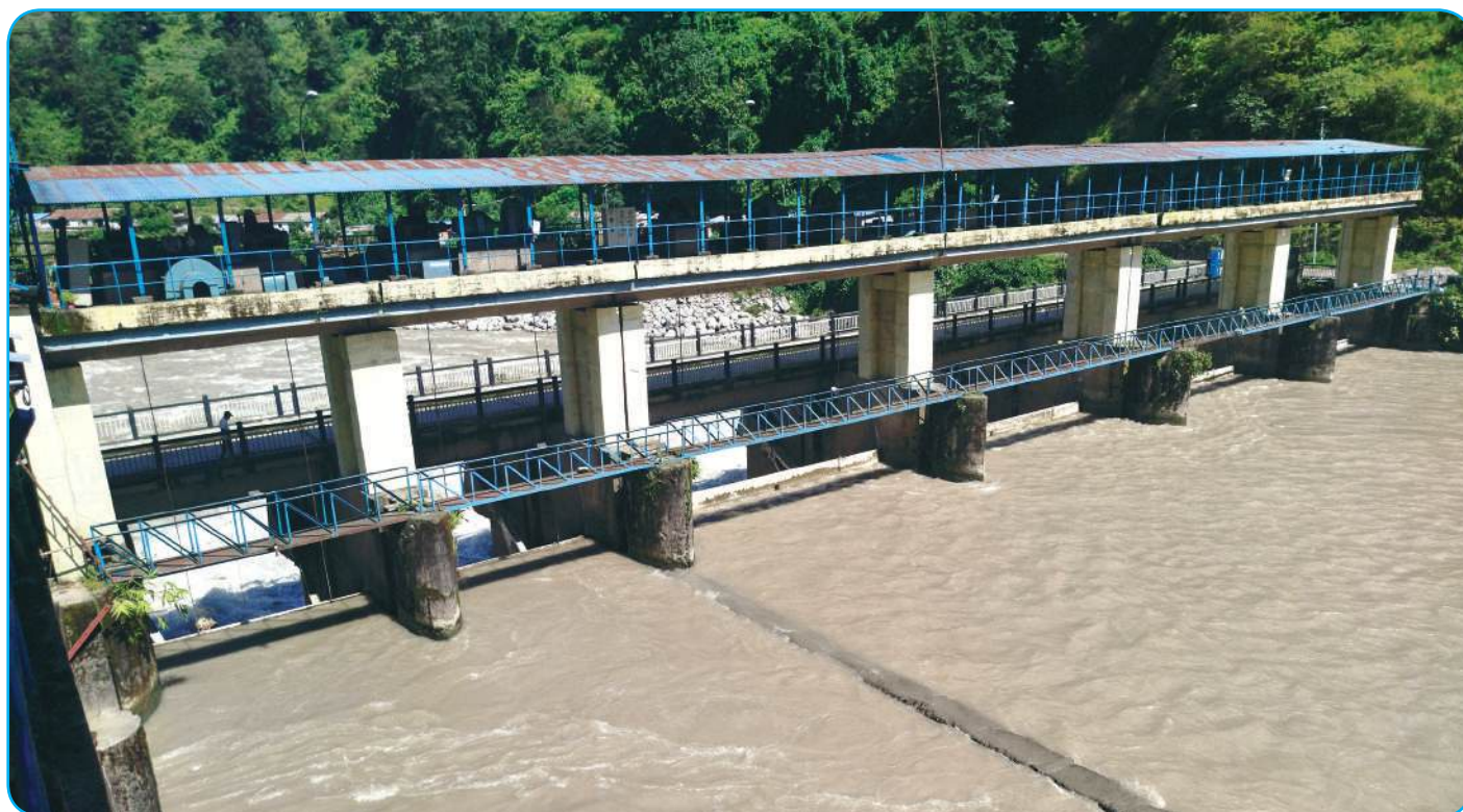
View of Damsite of Sunkoshi HPS
