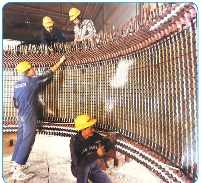
Generator Stator erection of 11kV winding (Marsyangdi HPS)
