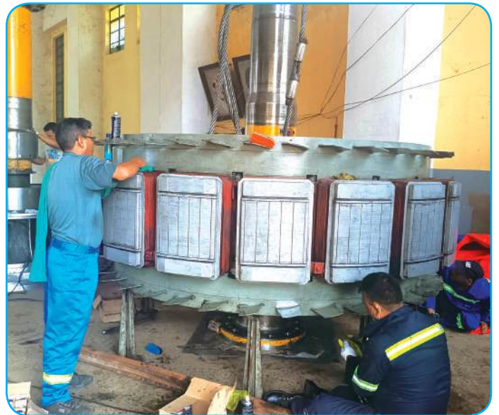
Surface protection work on runner
