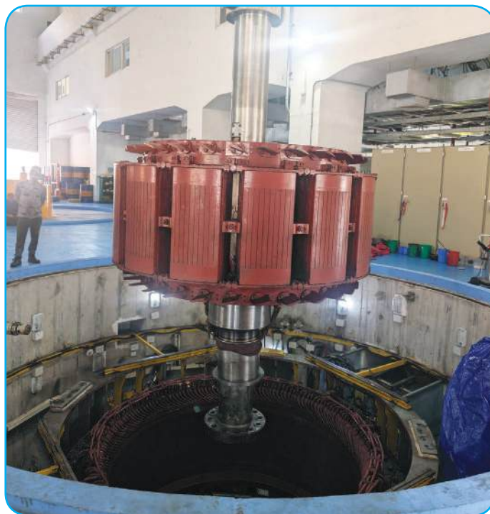
Rotor disassembly of unit 2
