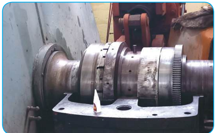
Repair of Thrust Bearing
