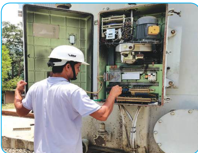
22.5 MVA Transformer TAP changer testing
