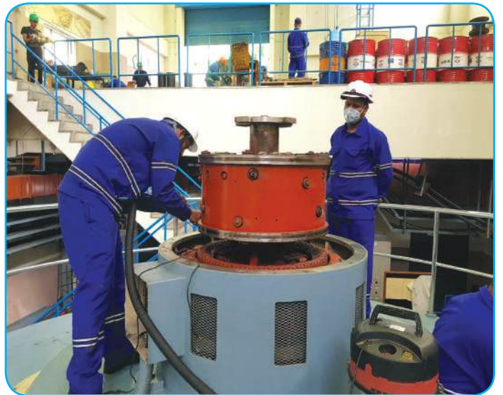
Cleaning & condition checking of Exciter
