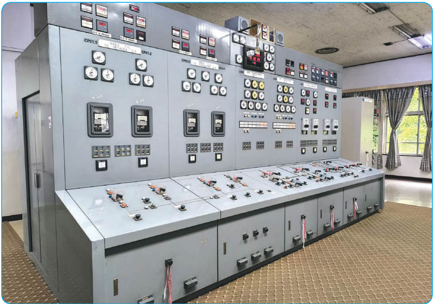
View of Control Room
