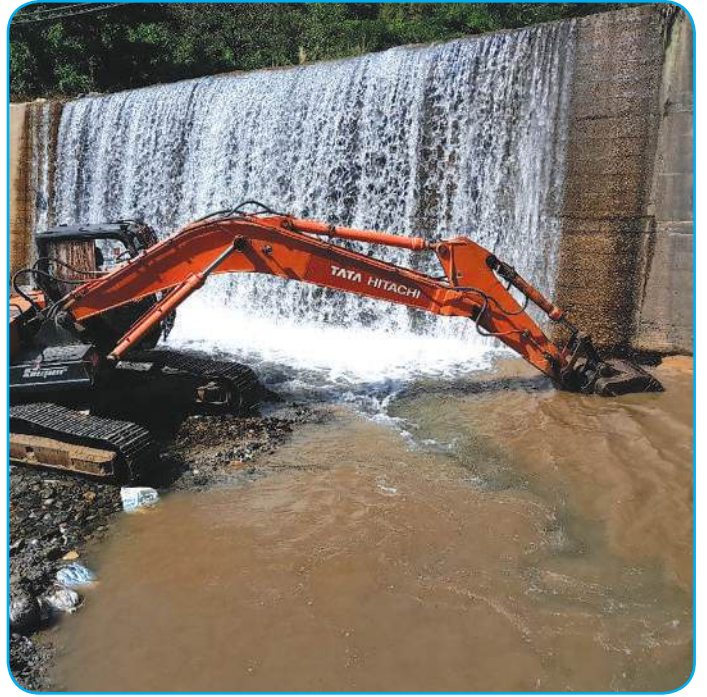
Debris cleaning at intake of Khanikhola
