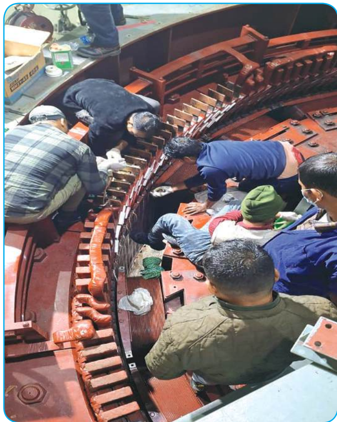
Replacement of new coils in Unit no. 2 R-Phase of Generator
