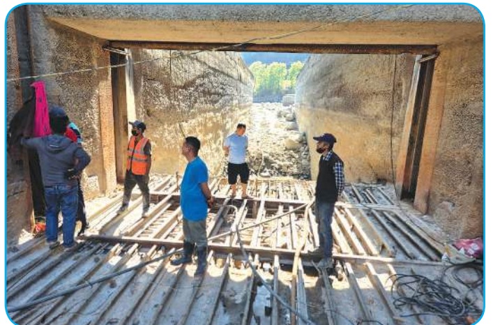
Gate undersluice Repair work
