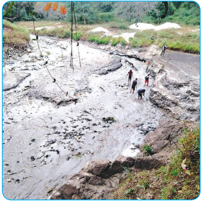
Deposit Debris Cleaning at Intake 3
