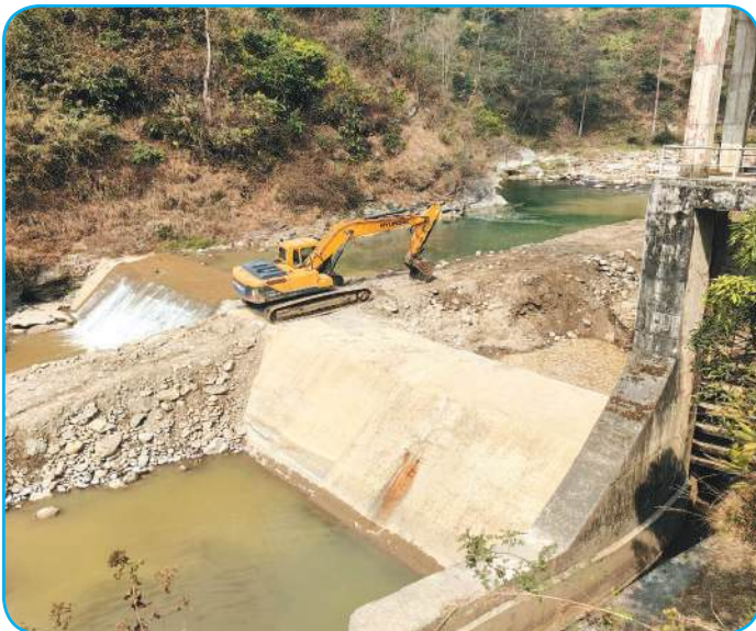
Construction of Cofferdam for Repair and Maintenance of Intake
