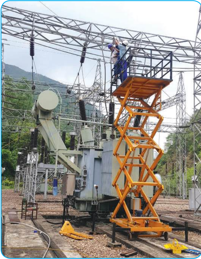
6.6 kV bus conductor maintenance
