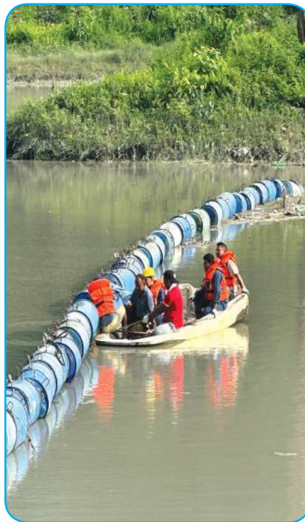
Clamping of Floating Boom Steel Rope
