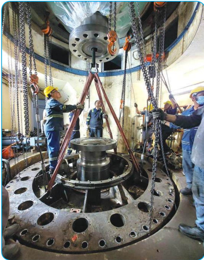
Unit No. 1 Overhauling works
