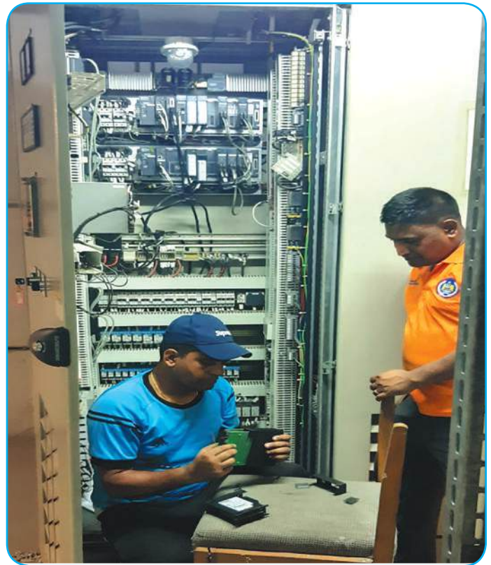
Governor panel installation work
