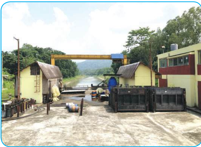
Intake Canal of CHPS
