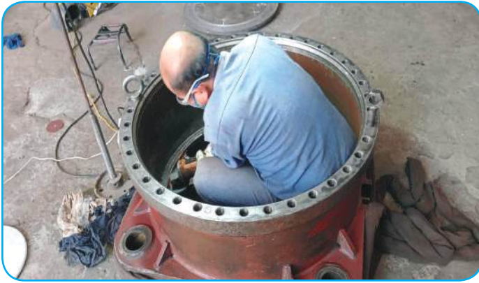
Piston Cylinder repair works for Unit No.2
