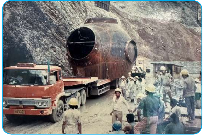
Transportation penstock Trifurcation during construction (Marsyangdi HPS)
