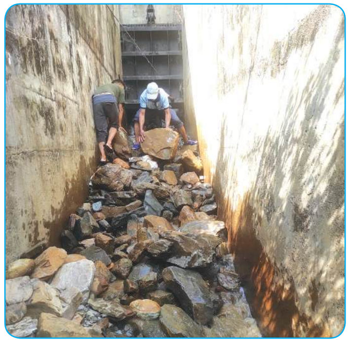
Chakhel Intake Debris Clearance and Gate Opening Work
