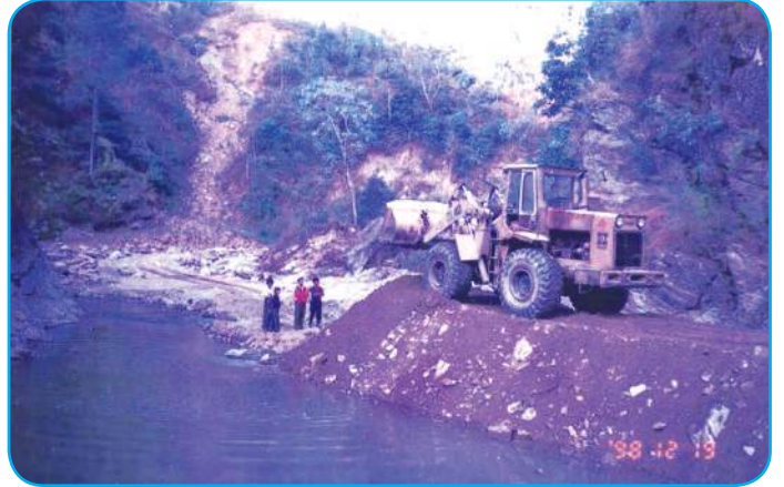
Coffer Dam of intake weir (Puwakhola HPS)
