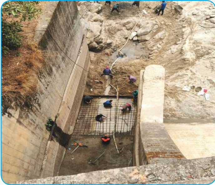
Repairing eroded chute of diversion weir gate of dam site
