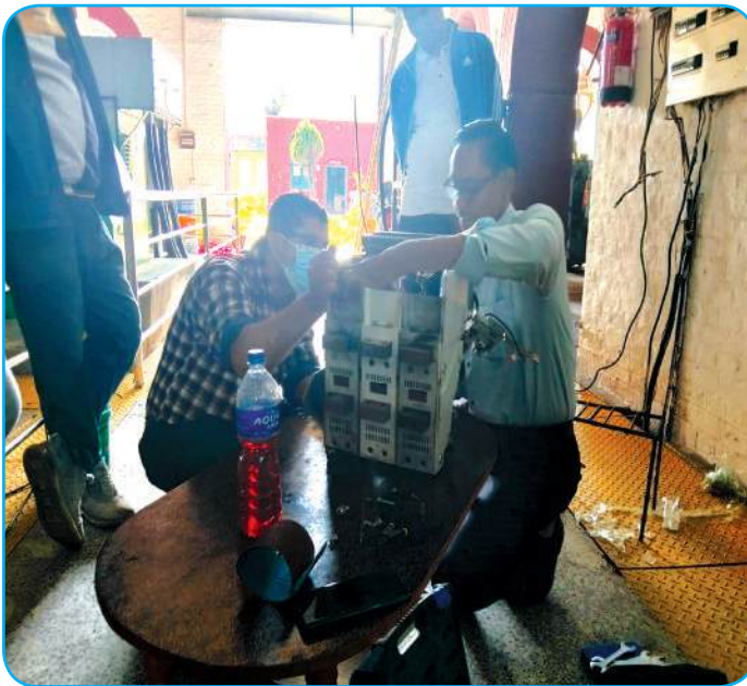
Repair of ACB 2
