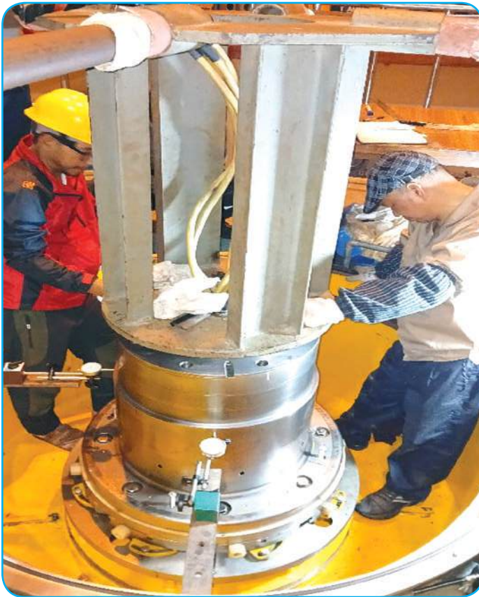
Manual rotating device used for shaft alignment of unit 2
