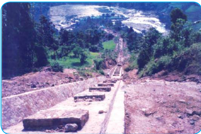
General view of saddles at penstock (Puwakhola HPS)
