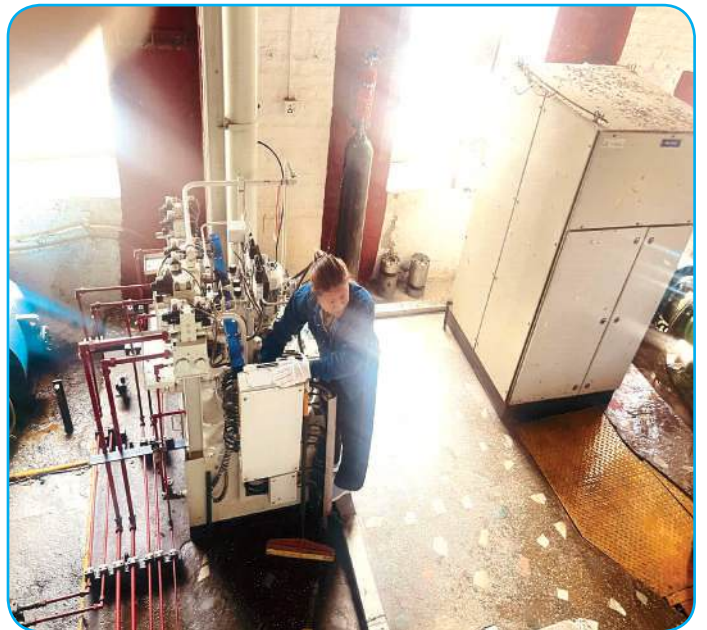
Maintenance of OPU 2
