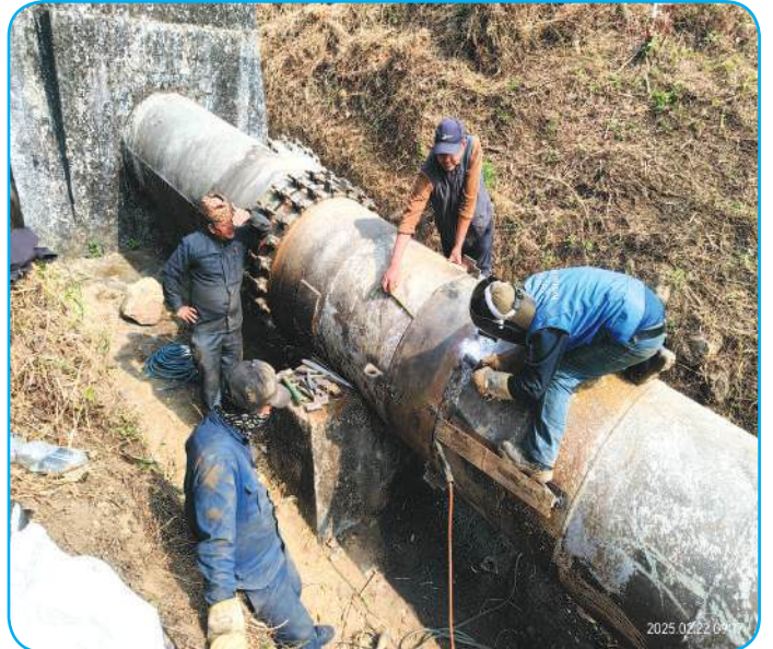
Penstock rectification works from Anchor Block AB#03 to AB#5A
