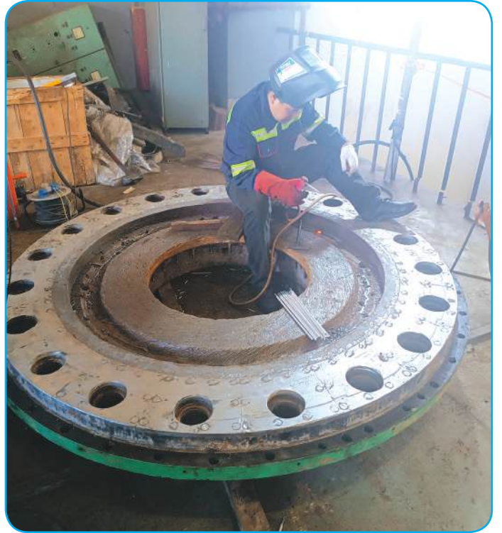
Turbine top cover repair works
