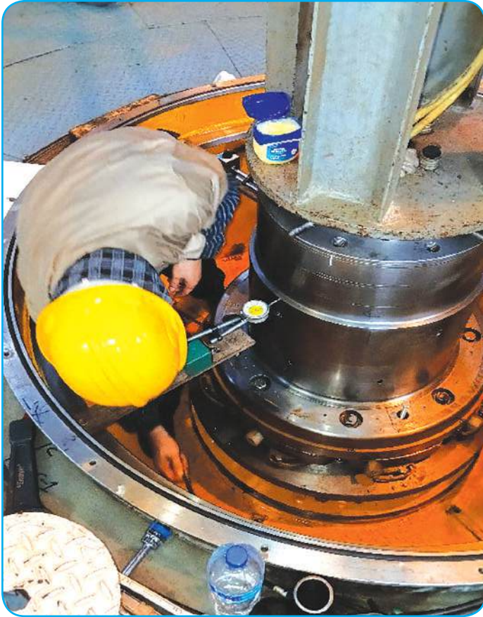
Unit no.2 Shaft alignment work
