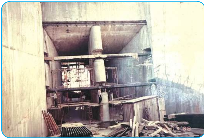
Installation of intake trash rack (Marsyangdi HPS)
