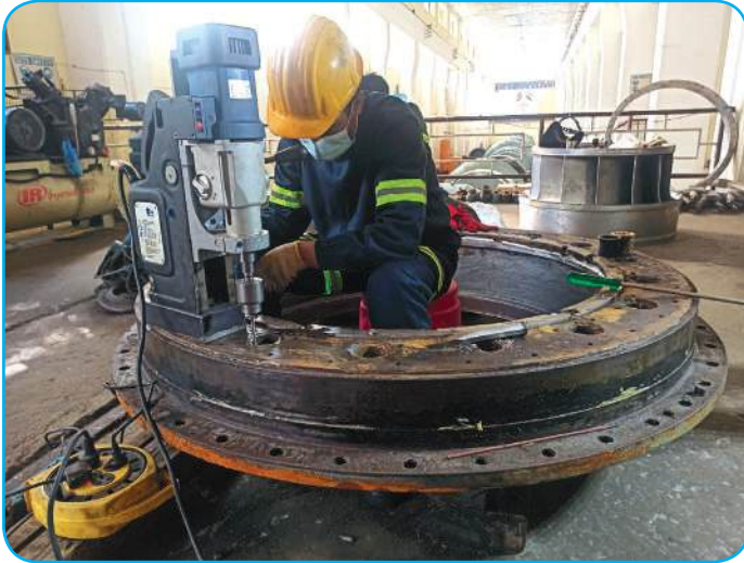
Repair of generator side cover
