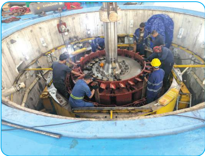
Unit 2 assembly works
