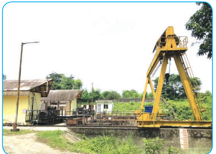
Gantry crane at intake
