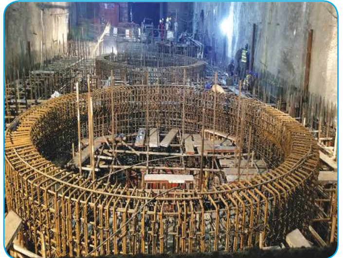
Generator Foundation works during construction (Upper Trishuli 3A HEP Project)
