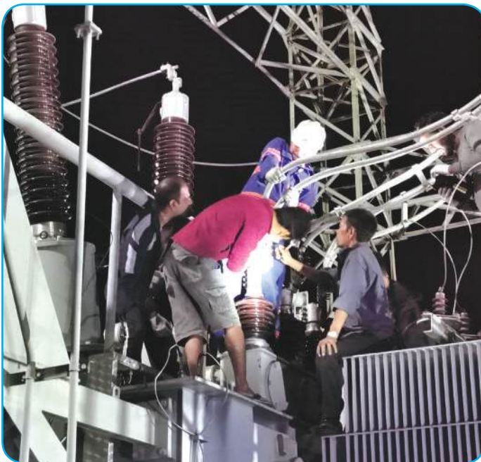
6.6 kV bus conductor maintenance
