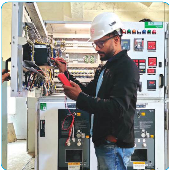
11 kV VCB relay changing work
