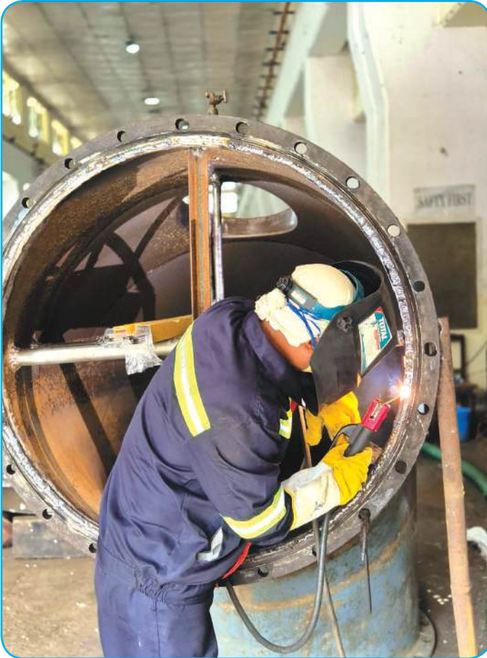
Draft Tube Bend Repair works
