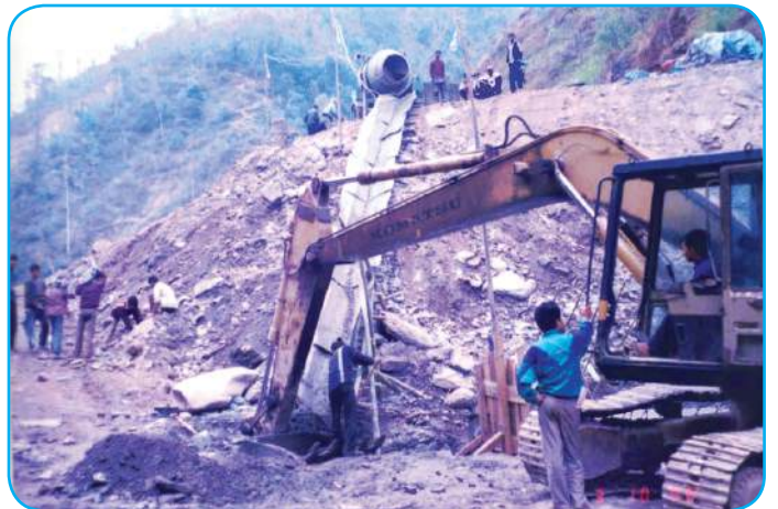
Intake gate installation during construction (Upper Trishuli 3A HEP Project)
