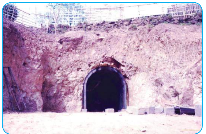
Portal of outlet Tunnel (Puwakhola HPS)
