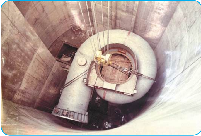
Lowering of Spiral Casing (Marsyangdi HPS)
