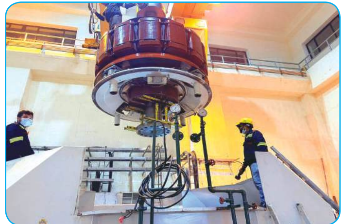
Rotor Installation works
