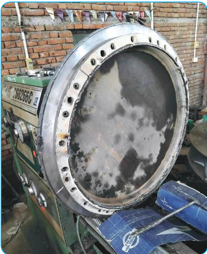
Machine Set up SS Split Ring repair works of Unit No.2
