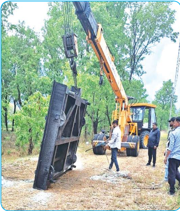
Gate Seal Replacement
