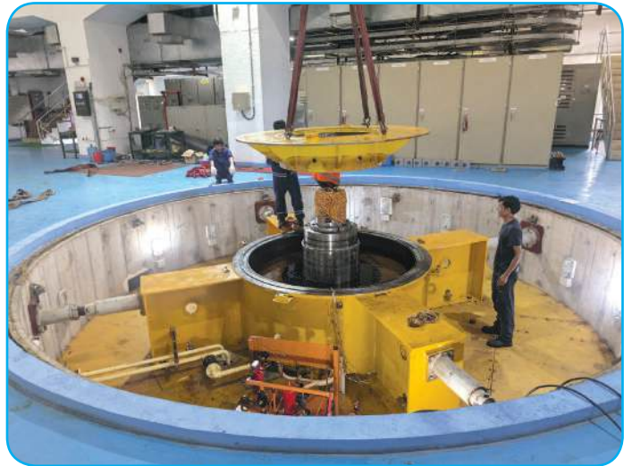
Lifting of upper bracket during overhauling
