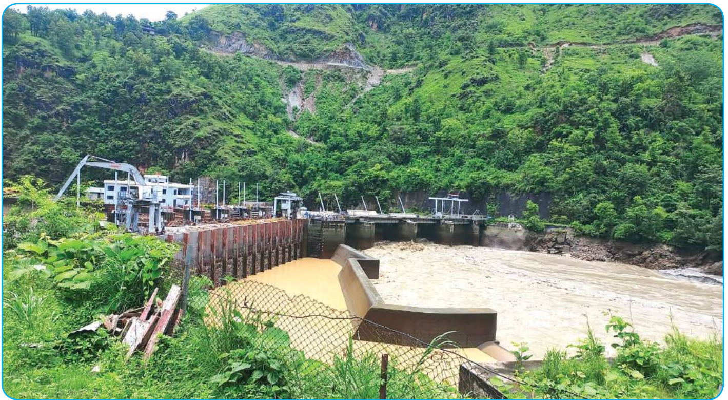
View of Headworks of Kaligandaki HPS
