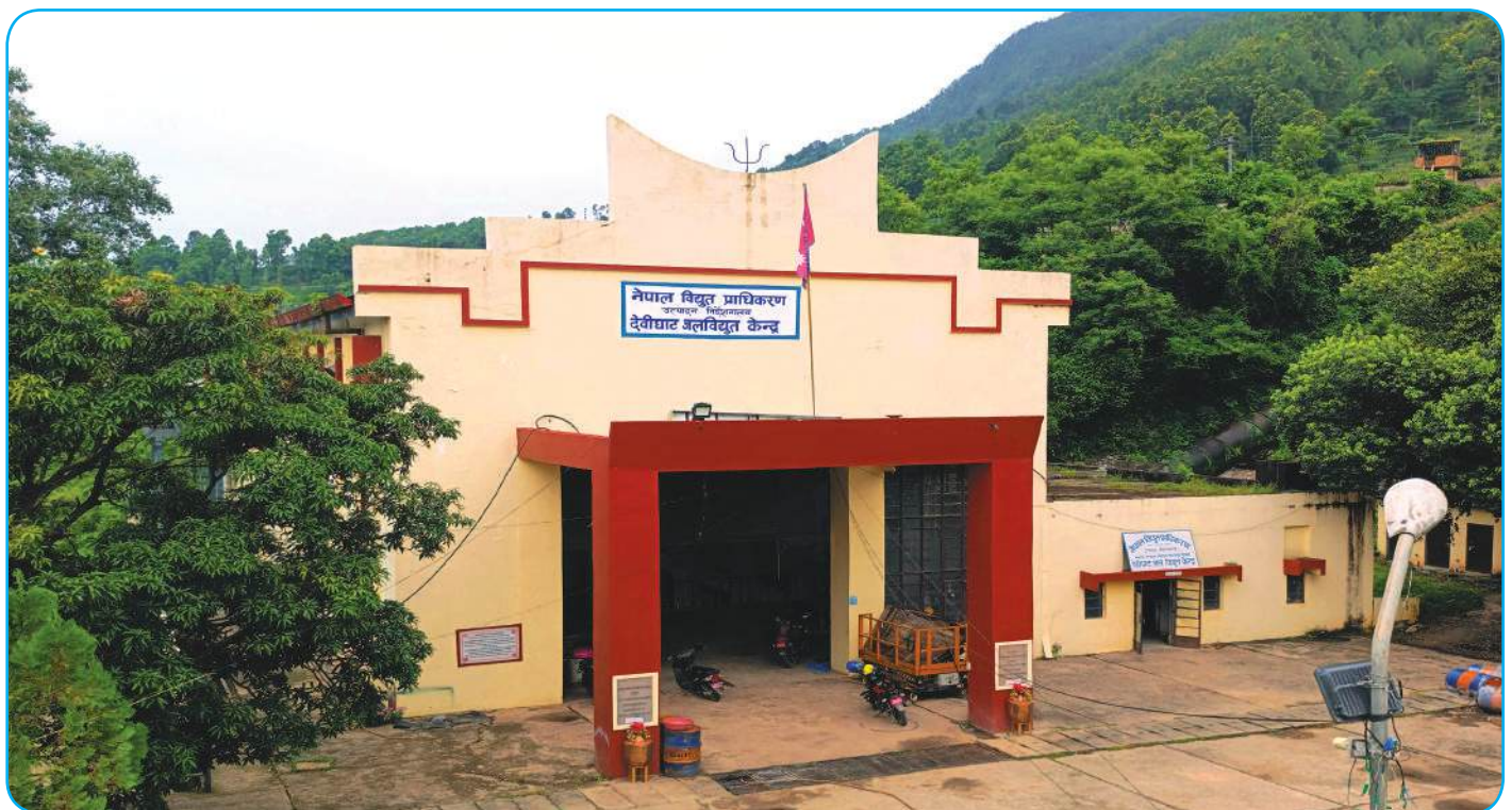
Powerhouse of Devighat HPS
