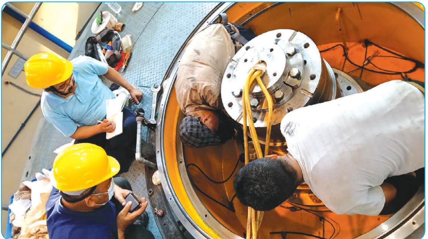
Unit No. 2 Shaft alignment work
