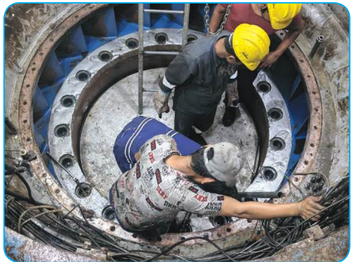
Removal of protective platings during unit overhaul
