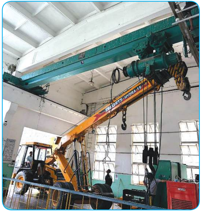
EOT Crane installation works
