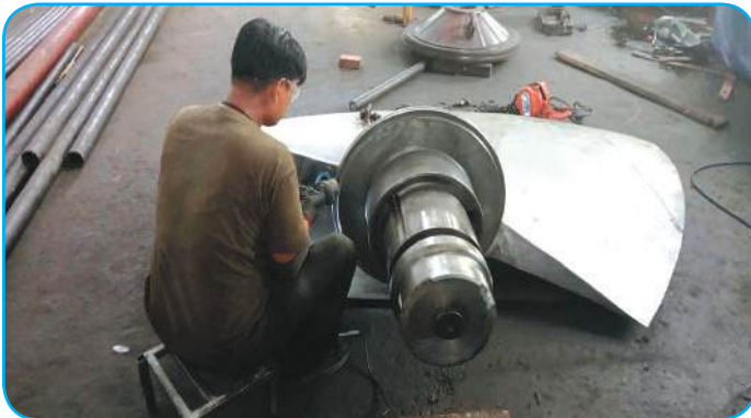
Runner repair works for Unit No.2
