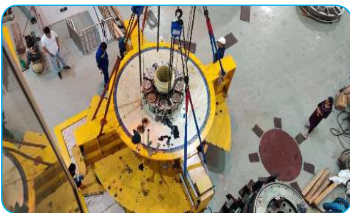
Lifting of generator bracket during overhauling
