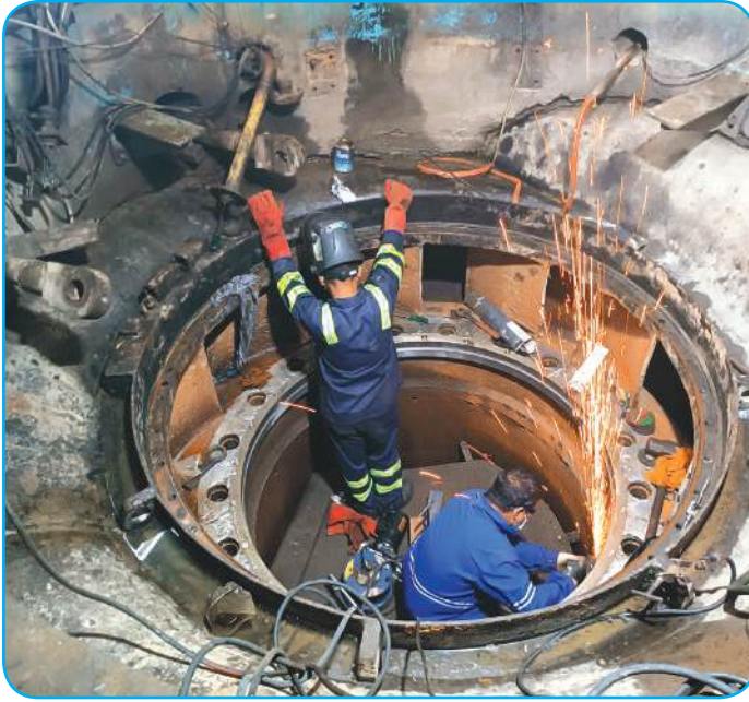
Repair of Draft tube
