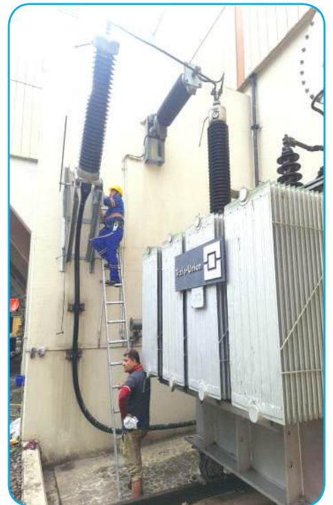
Cleaning of transformer bushing during overhauling
