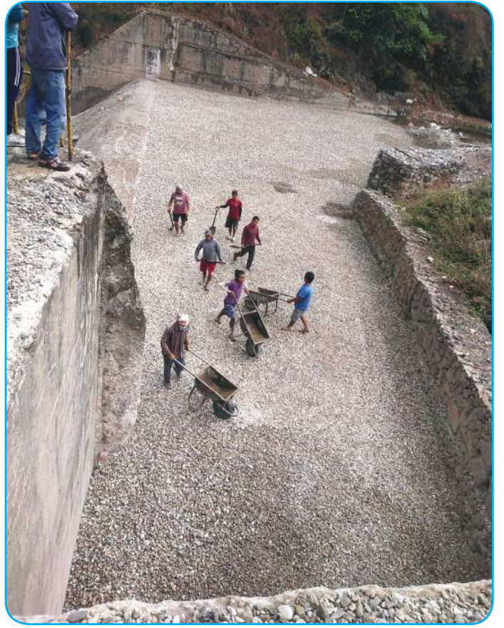
Filter Material replacement at Mandu Intake
