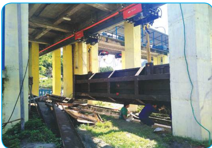
Installation of maintenance gates
