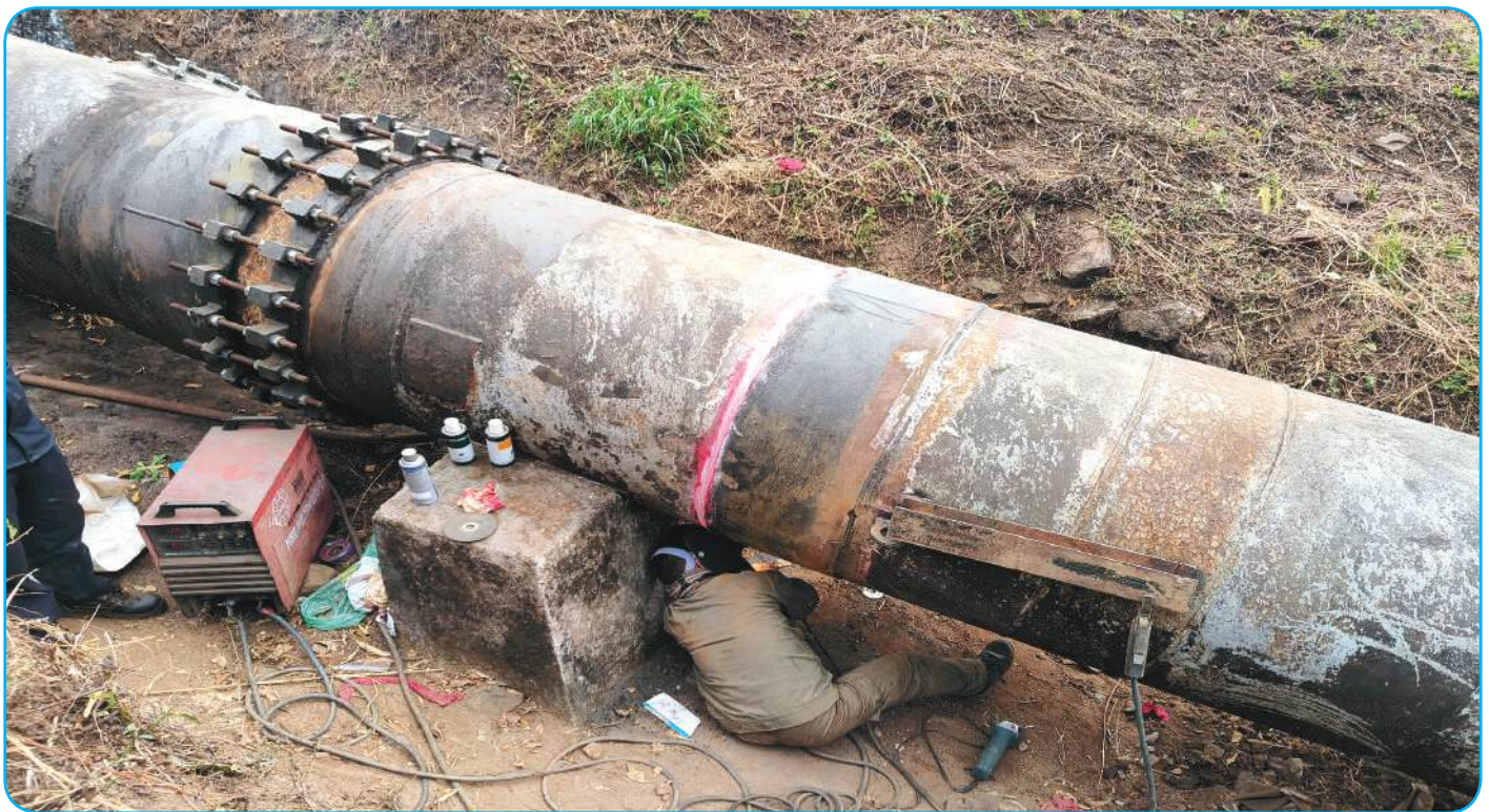
Penstock sectional rectification works
