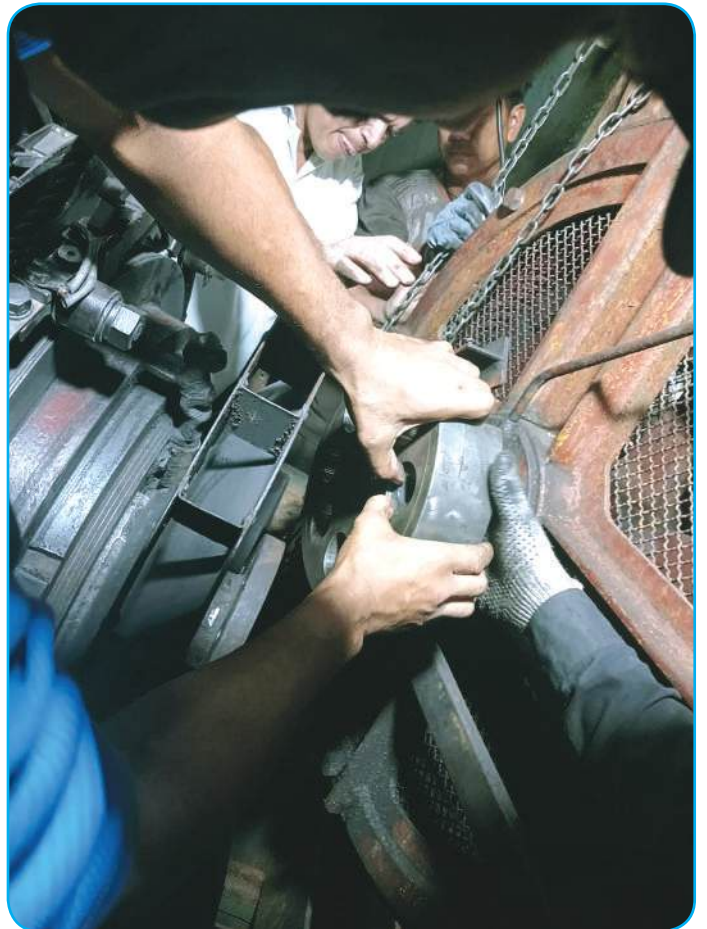
Installation of PMG Coupling for Unit No.2
