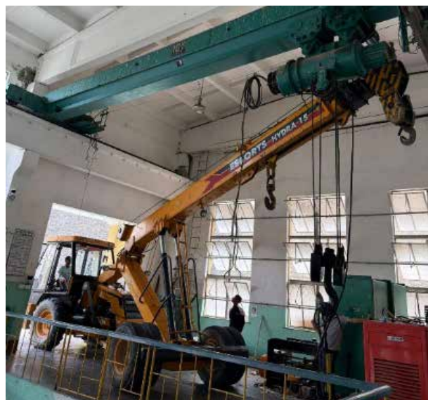
EOT crane installation works
