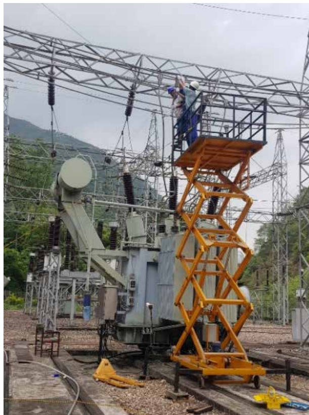
6.6 kV Bus conductor maintenance
