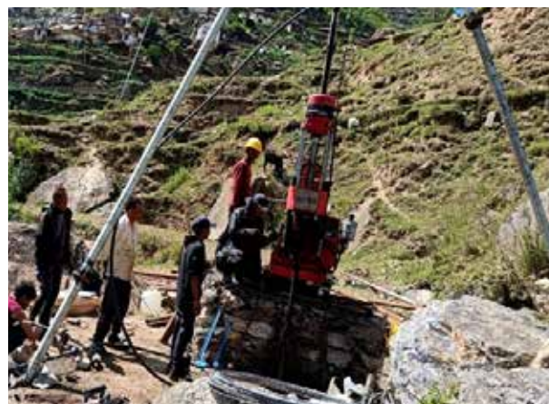
Core Drilling at JawaTila
