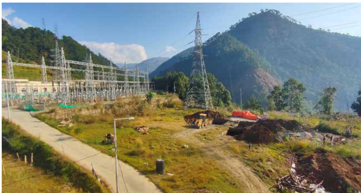
New Modi 132 kV Substation (with two Bay expansion & Foundation work)
