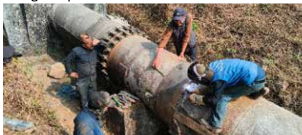
Penstock rectification works from Anchor Block AB#03 to AB#5A
