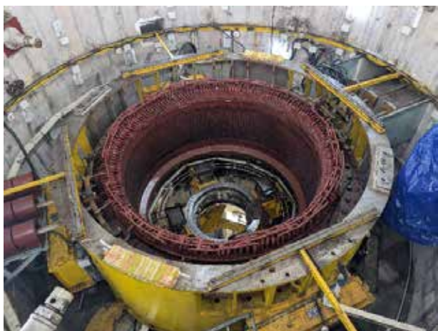
Stator of unit-2 during overhauling
