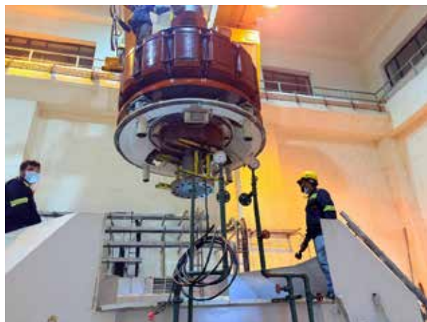
Rotor installation works
