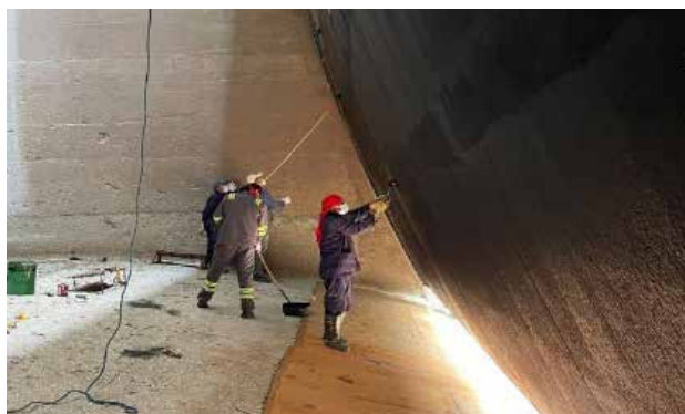
Radial gates repair works
