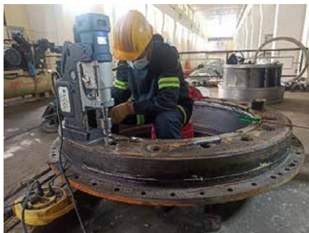
Repair of generator side covers during overhauling
